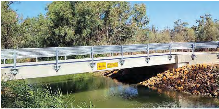
The Nelwart Street bridge, opened in April 2025. PHOTO: RIT
