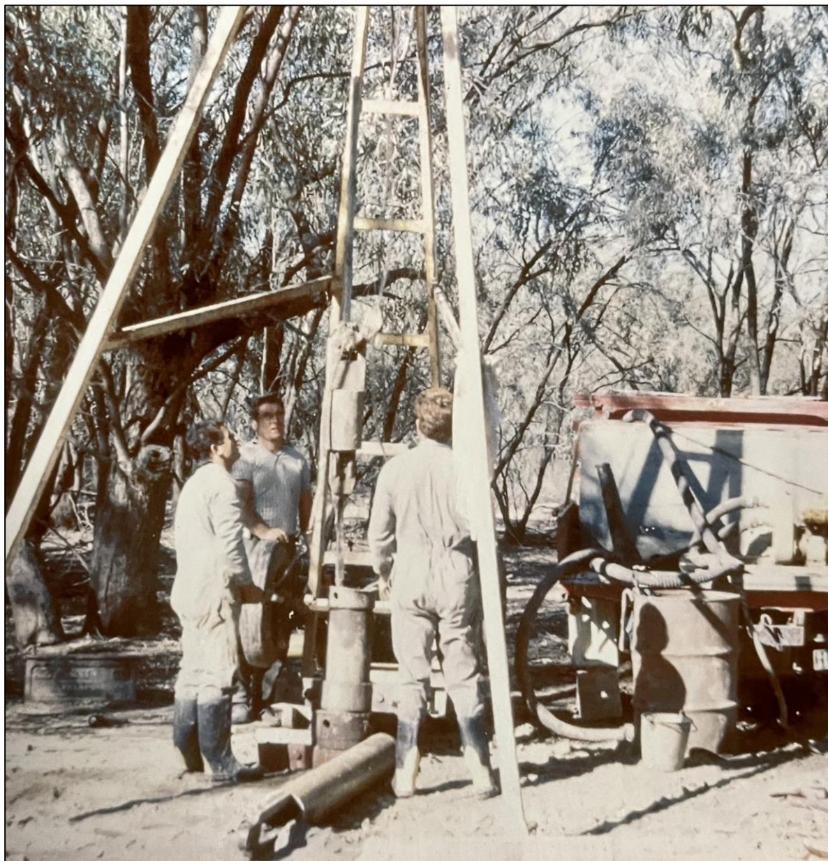
1963- 5 Initial investigations: boreholes and bitumen testing
