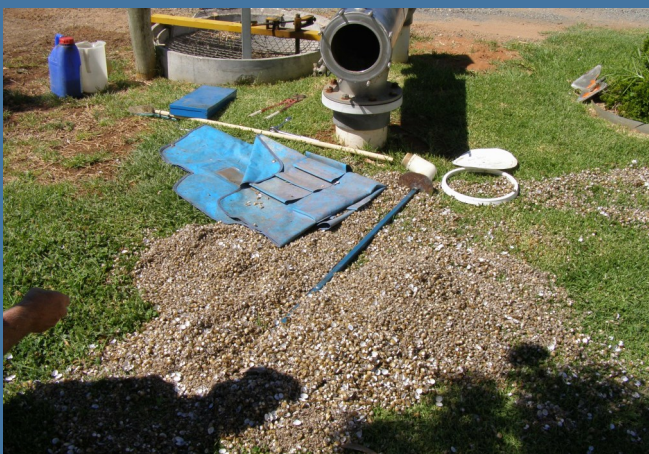
Shells removed from an Irrigator's filter
