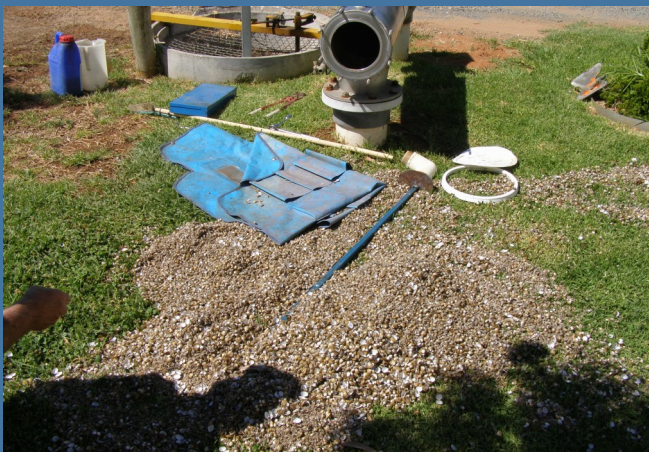
Shells removed from an Irrigator's filter
