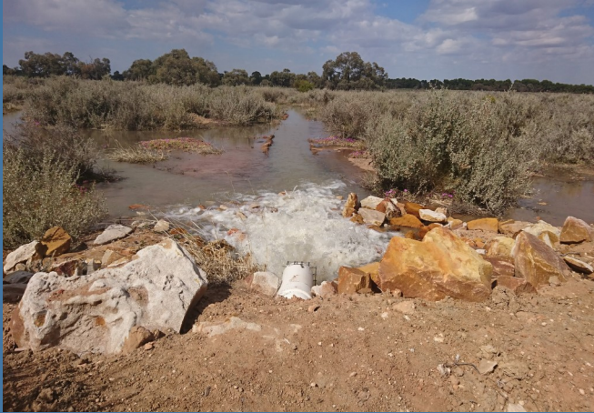
Environmental watering has helped with the flushing of fouling growths from pipelines
